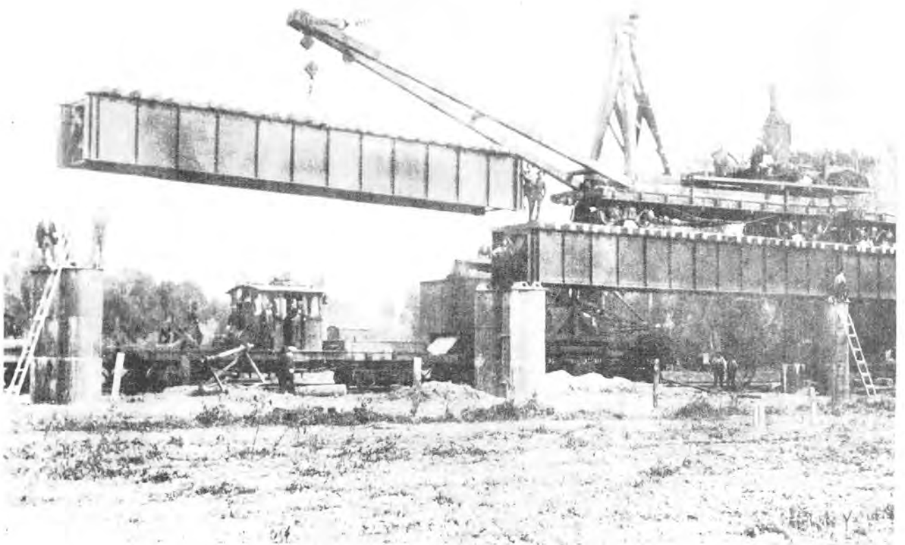
"OLD MAUDE" --- Motor 701 --- and crane 1225 hard at work on Butte Slough Bridge, Colusa Branch, on November 1, 1919; this shows 701 with original Baldwin trucks.
