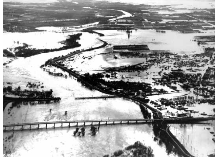
1955 FLOOD – 10TH STREET BRIDGE IN FOREGROUND, 5TH STREET BRIDGE WASHED OUT
