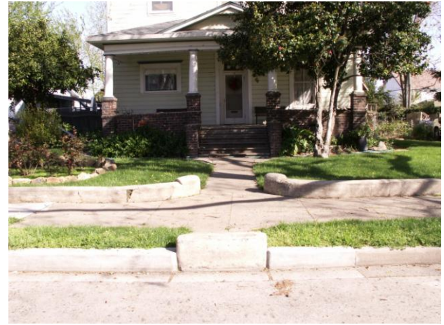
View showing the concrete border around the property and also the carriage step
